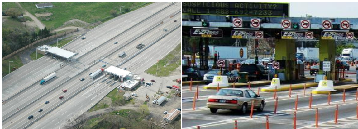
Figure 6 : RFID approaches: I-Pass mixed ORT/Cash toll plazas (Illinois) and E-ZPass specific lanes in toll booths
